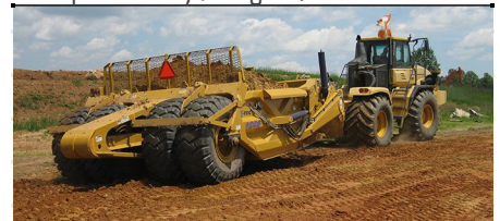
Topsoil / Manitoba, Canada
